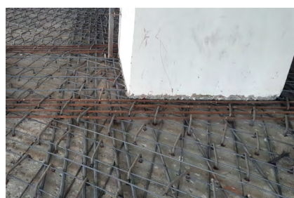
c) Slab strengthening
