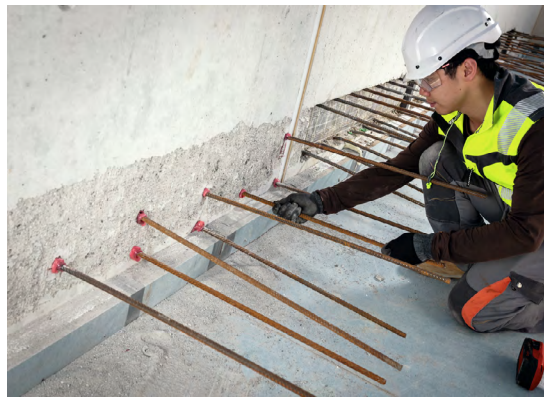
b) Slab-to-wall connection
