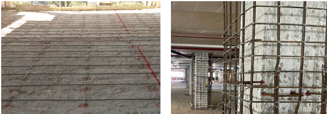
g) Slab shear-friction overlay
