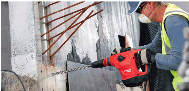
Fig. 9.4: Hammer drilling (HD) tools
