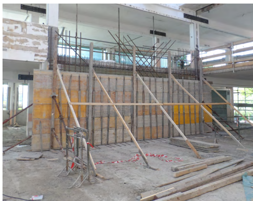
b) Interior walls
