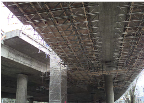
c) Increasing bridge girder thickness
