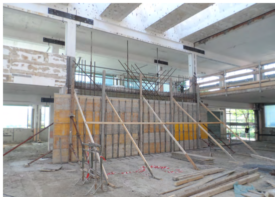
e) Shear wall addition
