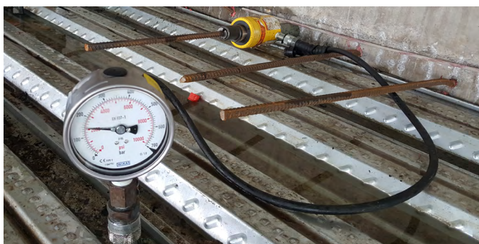
c) On-site inspection of post-installed rebars installation
