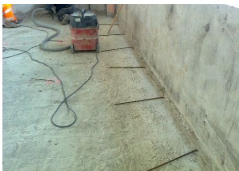
b) Connection of overlay to perimeter walls
