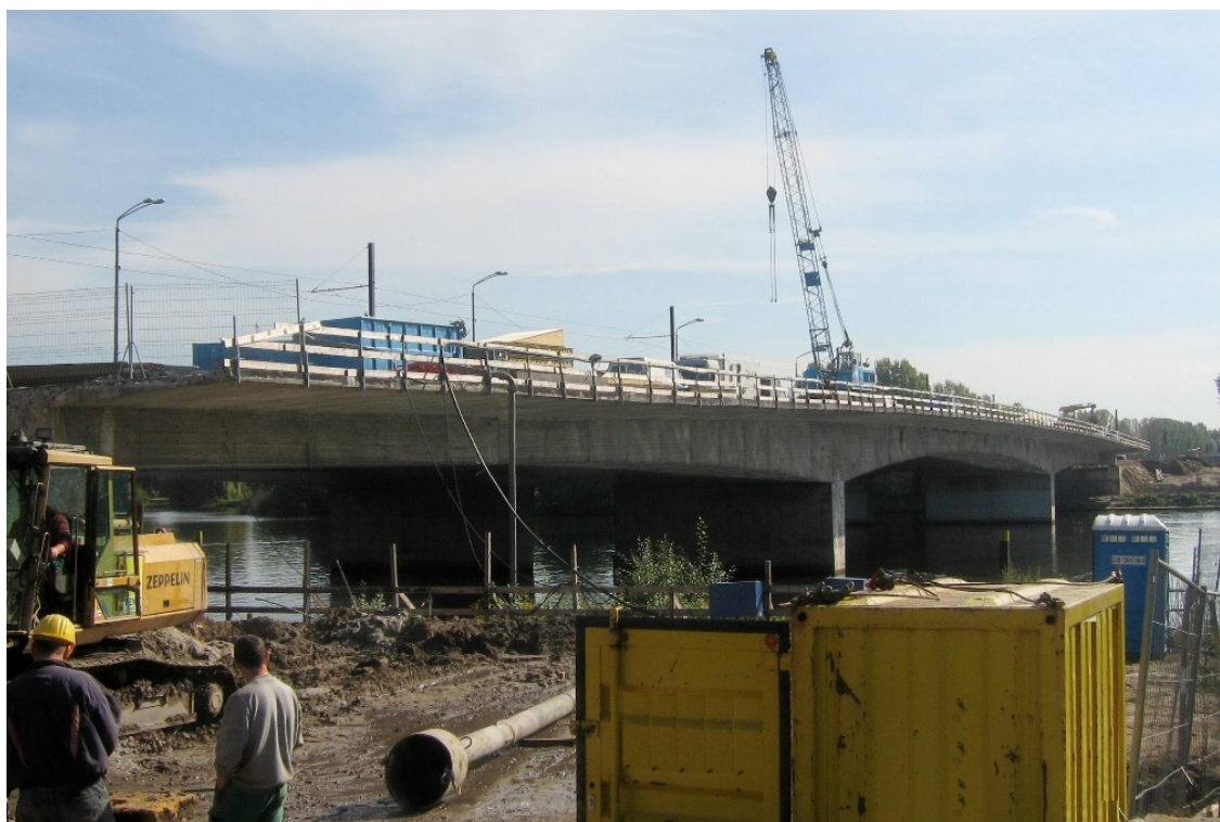
a) The bridge to be restored
